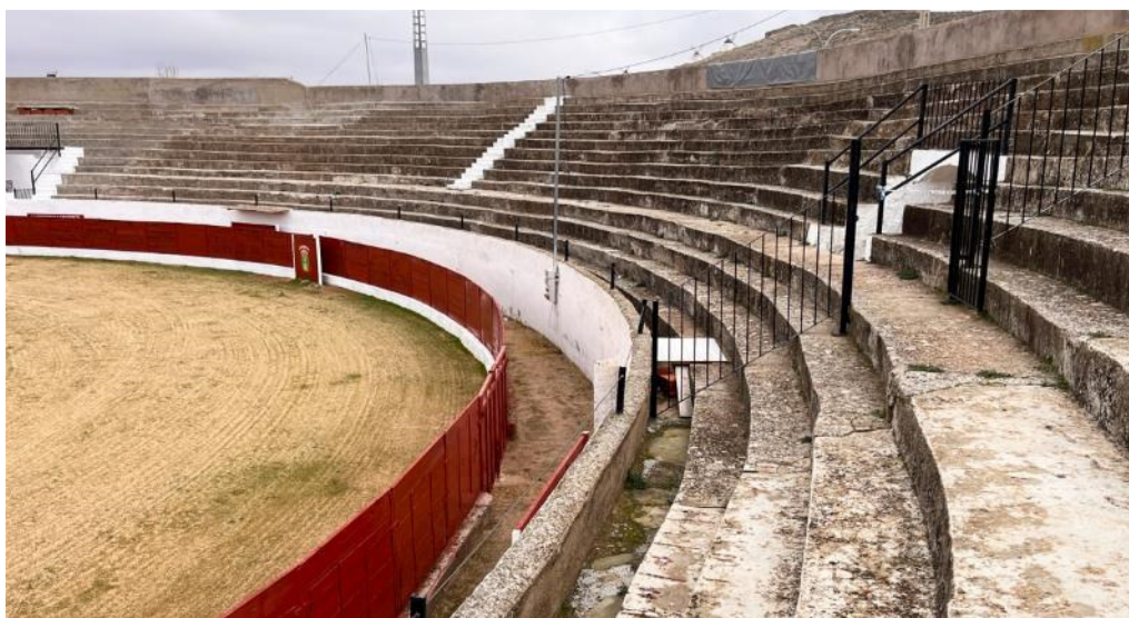
Vista general tendido sureste (sol)
